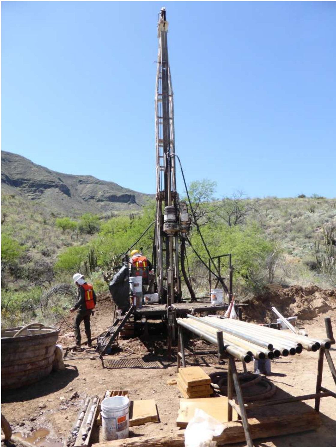
Figure 10.1: 2015 Drill Rig Producing NQ Drill Core
